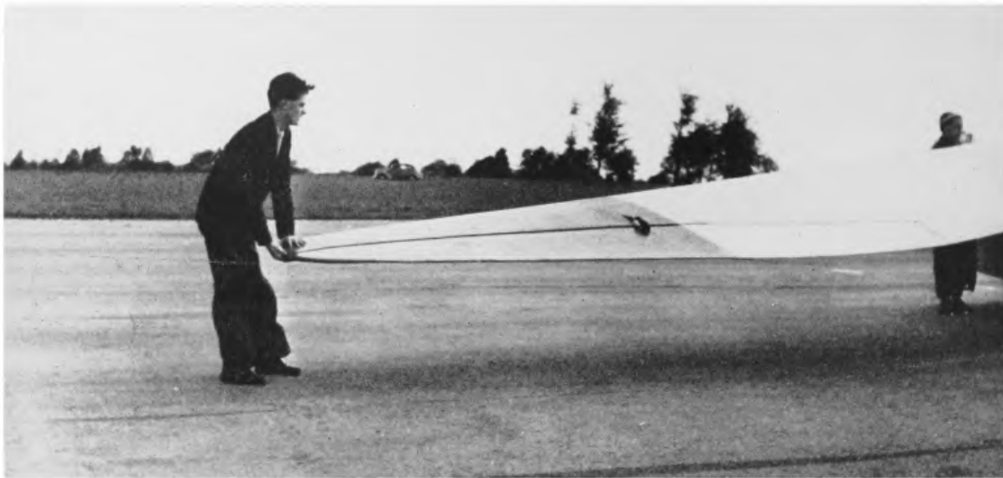
26. The first thing the new member has to learn is how to handle a glider in a wind. Gliders can fly in very strong winds quite safely, but on the ground they will quickly blow over if not treated properly. When the wing is into wind it must be held low, or put on the ground and kept there with a heavy weight such as a tyre.
