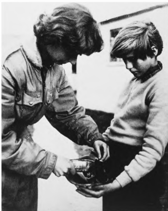
20. Afterwards, if the pilot wants to keep the barograph record of his flight, it is fixed by dipping it in a solution of shellac and methylated spirits. This prevents the smoked paper from smudging the traced line.
