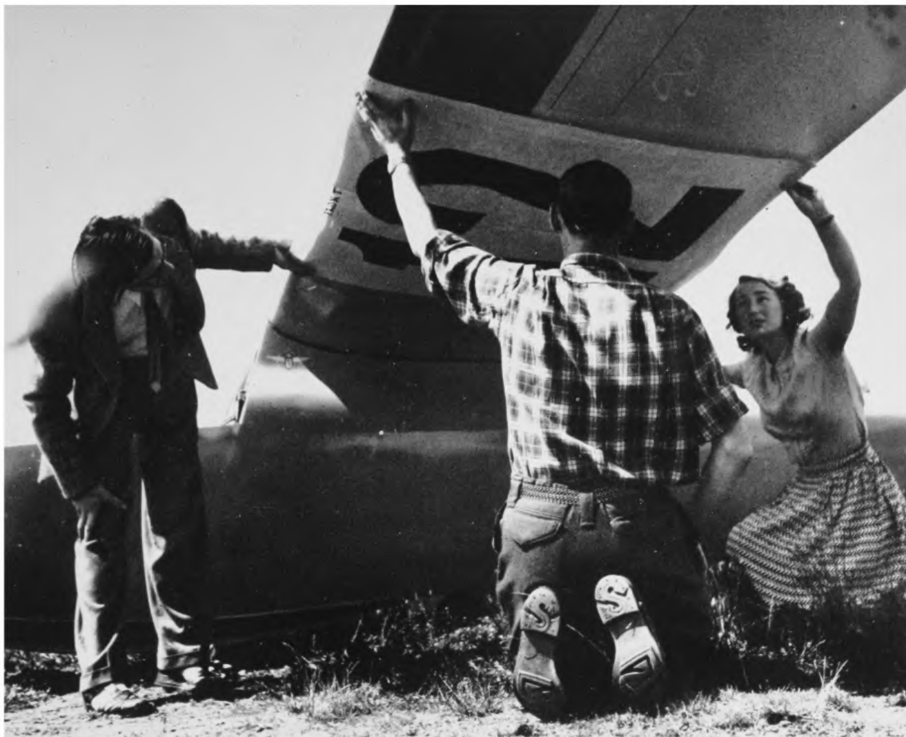
110. Each glider has a competition number. These are fixed on the underneath of the wing and on the rudder, so that the glider can be identified from the ground at turning points.
