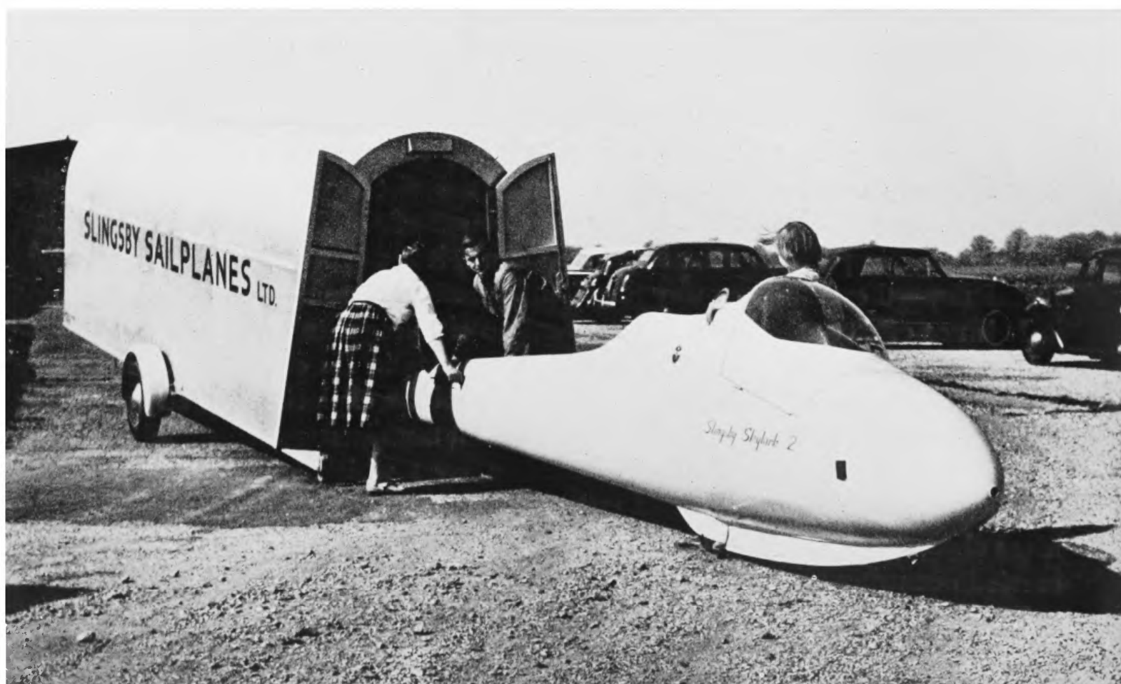
2. This is the trailer in which Philip tows his glider to the club, and inside it fits the whole glider. Elizabeth and Bob help Vanessa out with the fuselage, being careful not to damage the top of the rudder on the doorway.
