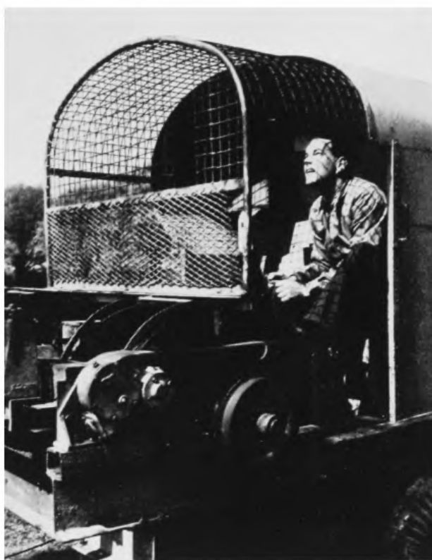
58 (left). Winching is one of the most complicated jobs in a gliding club, although liked by those sufficiently mechanically minded. New drivers must be taught carefully, as the lives of the glider pilots are in their hands. Tom, the expert, stands by while the pupil concentrates on taking up the slack in the cable without a jerk.
