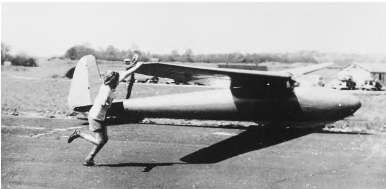
56. While the glider is gaining speed, the wing must be held level, by someone running fast on the wingtip. Fortunately this is usually only a matter of a few yards.
