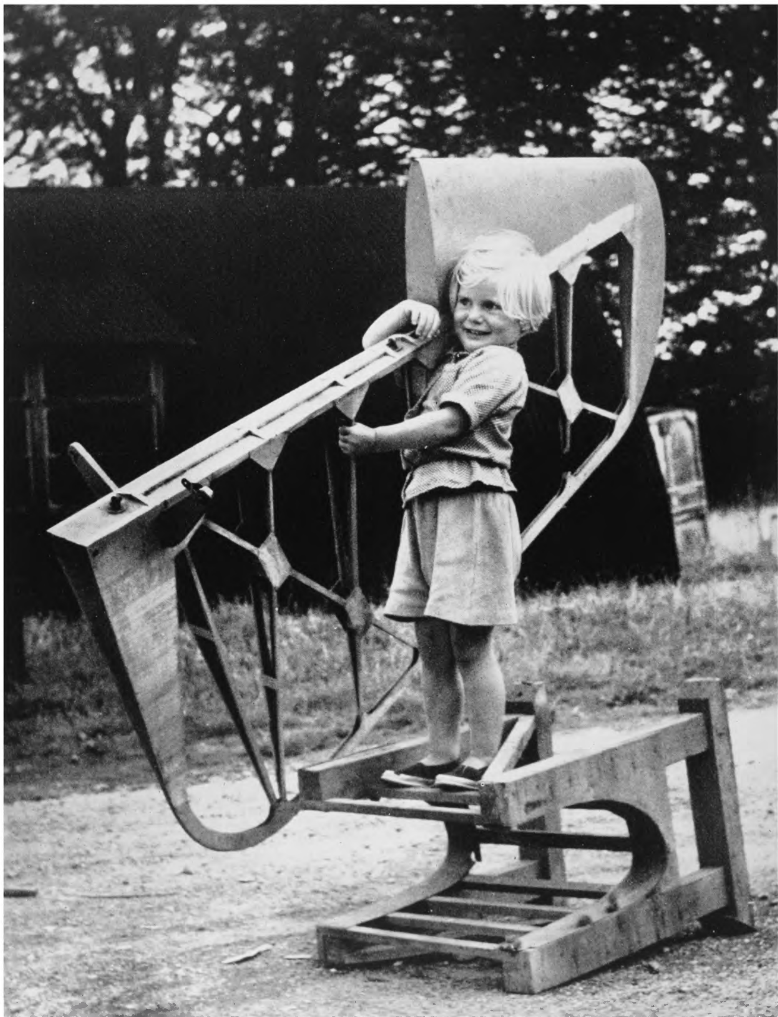
Gliders are made with great care to be light yet strong. Janet, aged just 3, is holding the rudder of a school two-seater—and it wouldn't really matter if she dropped it.
