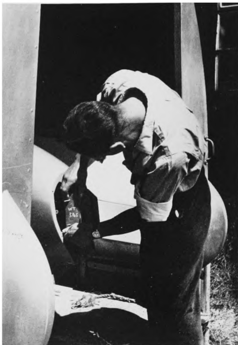
30. The centre of gravity, or the balance, of the glider is determined by the pilot's weight. If he is very heavy the glider will tend to fly nose down, and if he is light it will tend to fly nose high. If the pilot is too light, and less than the permitted minimum for the particular aircraft, the pilot must put more weight in the nose before taking off. Here Steve is putting ballast into his Sky.
