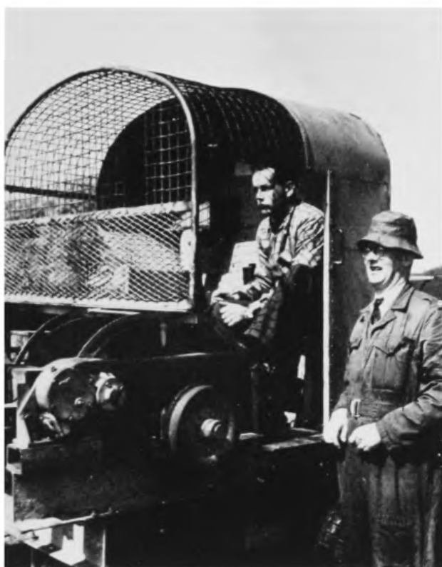
58 (left). Winching is one of the most complicated jobs in a gliding club, although liked by those sufficiently mechanically minded. New drivers must be taught carefully, as the lives of the glider pilots are in their hands. Tom, the expert, stands by while the pupil concentrates on taking up the slack in the cable without a jerk.
