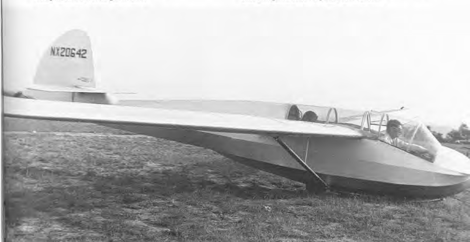
The prototype SGS 2-8 sailplane owned by the 'Airhoppers' Club. The nose was later lengthened. On this aircraft there was no window below the wing. This was added to later aircraft.
