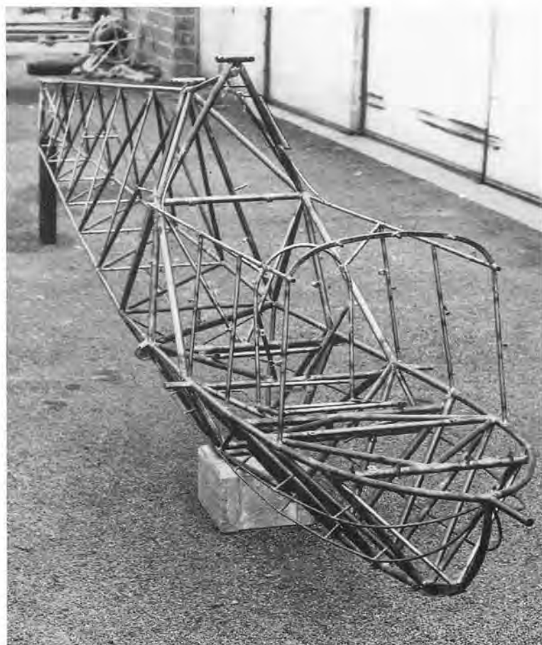
ABOVE: The welded fuselage frame of the SGS 2-22.
