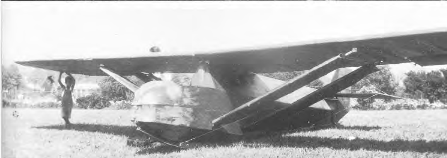
TOP: Paul Schweizer in the SGP 1-1 Primary. Note the rope on the tail for holding the glider back during the first phase of shock-cord launching.
