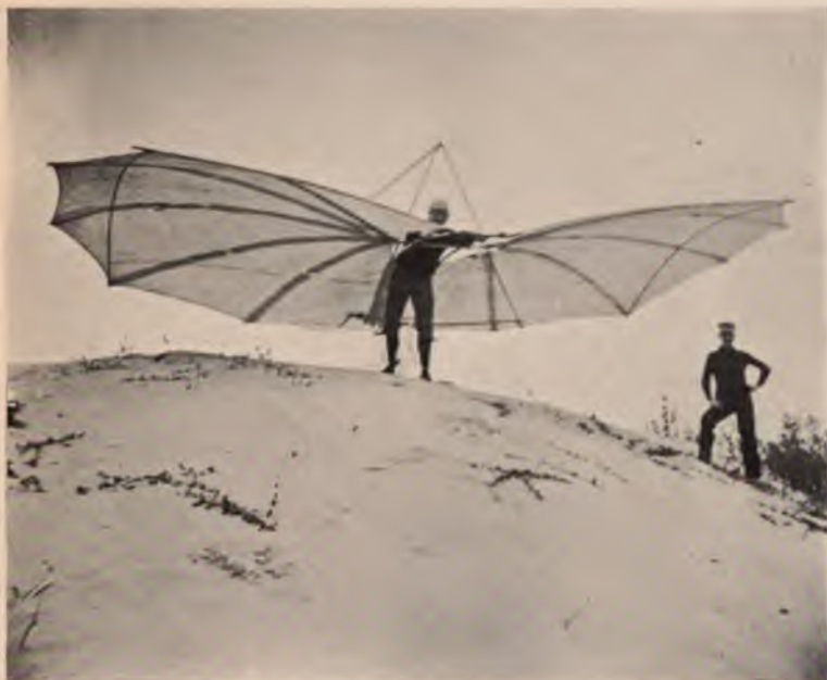
Fig. 1. — GLIDING MACHINE. p. 33.
